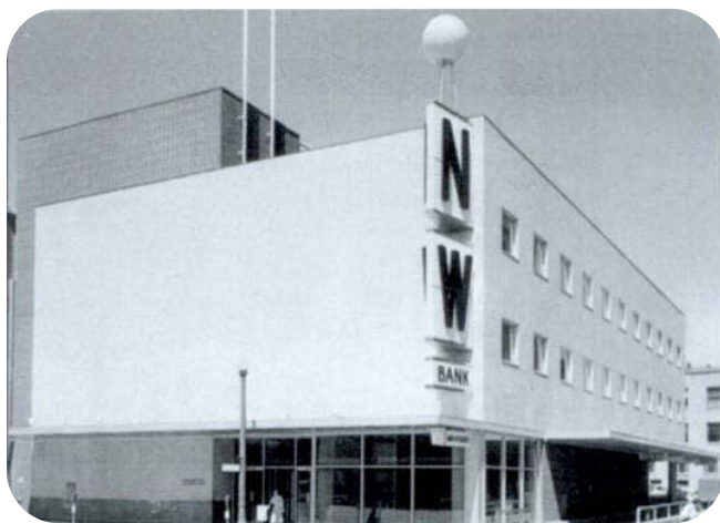
Northwestern National Bank, located at 15-21 2nd Street SW and built in 1957, is an example of the International style of architecture. Source: City of Rochester
