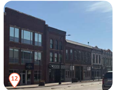
9 Though modern, the newer development beginning at 316 Broadway and north acknowledges the district's scale and style
