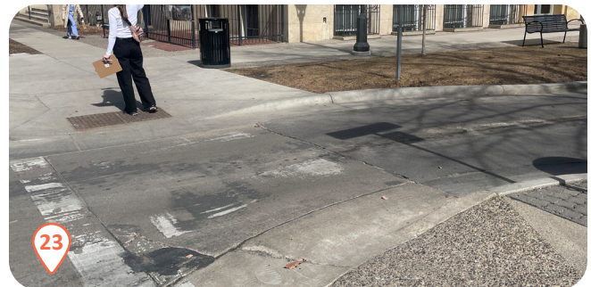
Crosswalk improvements will lend to a better feeling of safety and comfort crossing roadways
