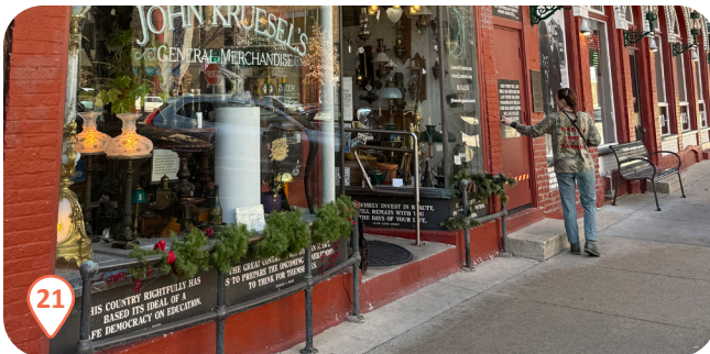
Steps up to businesses are barriers to some, and back-of-house entries feel unsafe and too far a distance to travel
