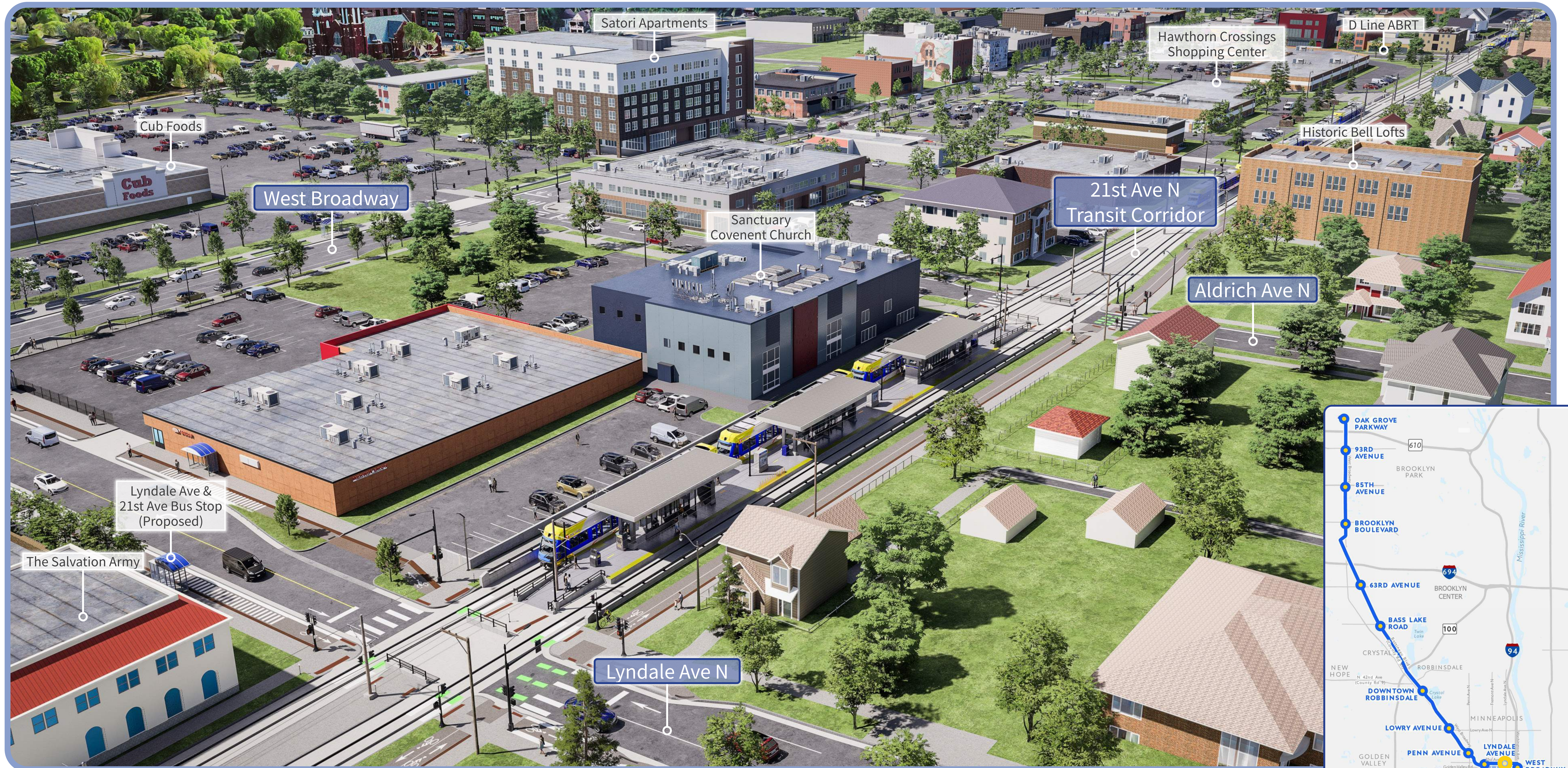
Lyndale Avenue Station looking southwest
